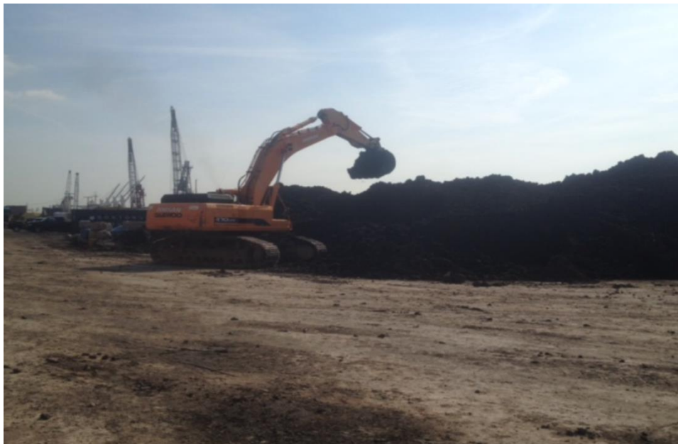
Figure 4 Mixture of displaced materials and Portland cement is placed in piles to dry out the moisture
